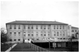
St Anthony's Home, Kew, buildings [rear]
