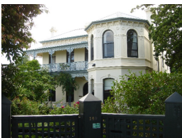
Rathgar, 149 Victoria Road, Hawthorn, Boroondara City
