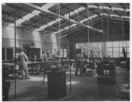
New woodwork shop at Bayswater Youth Training Centre, constructed entirely by staff and trainees
