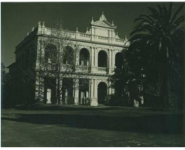
Blackhall, 26 Sackville Street Kew
