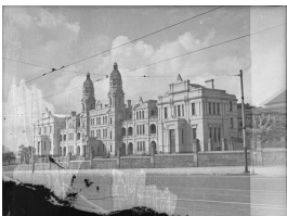
Deaf, Dumb and Blind Institute building, Darlington
