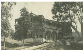
Green Place on the Swan River, Mosman Park
