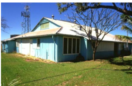
Pine Creek Repeater Station
